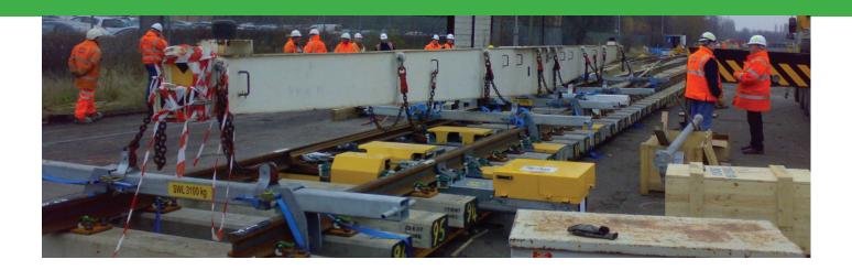
OUR S+C CROSS BEAMS are designed to be pre-fitted to S+C panels prior to shipment. Once on site they can be swiftly attached to a spreader beam ready to lift the panel into place with the minimum of wasted site time.
