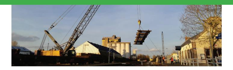
HOOK PANEL HANDLERS are designed for single-point lifting of track panels. A key feature of this product is that, like the Hook Lift Beams shown on page 6, these do not require a hydraulic or other power source.
